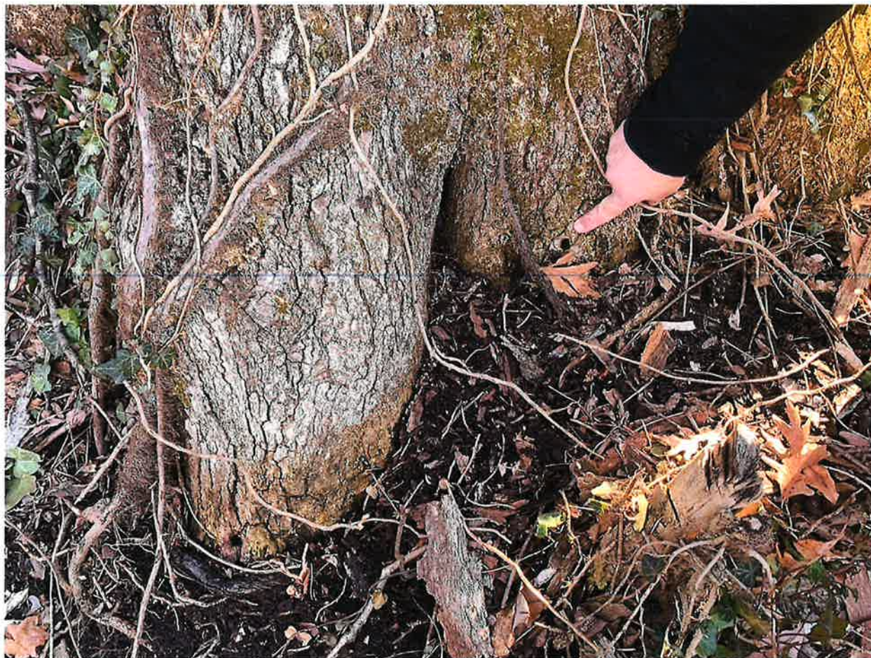
Image 3. Bore holes in Tree T39 that Mr. McCully and Mr. Tan observed during their February 8, 2022, site visit. Photo taken by Mark Tan on February 8, 2022.
