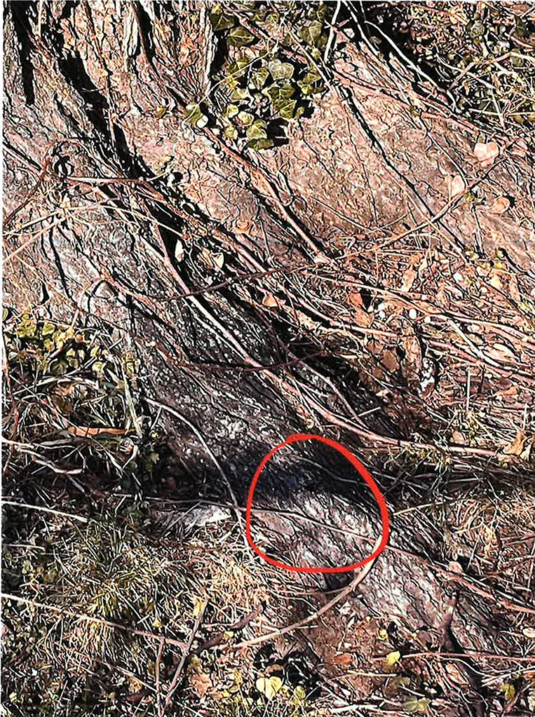
Image 13. Bore hole observed in the root flare of Tree T1 at 2440 Shannon Pl., SE. Photo taken by James Biddle on February 16, 2022.
